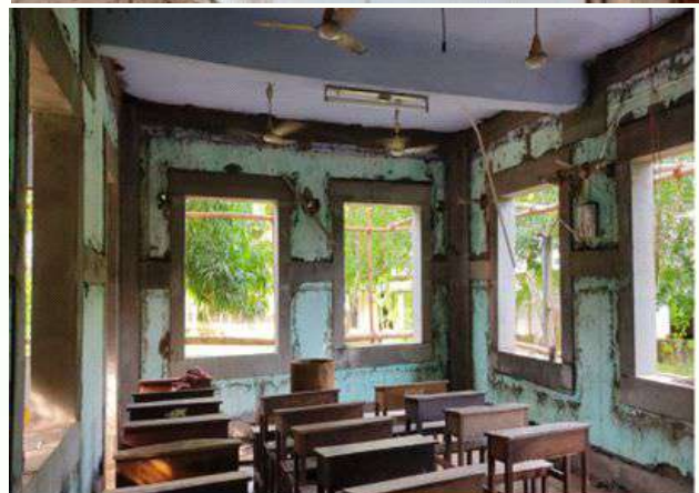
Retrofitting of Melaghar Girls H.S(+2) School, Tripura
