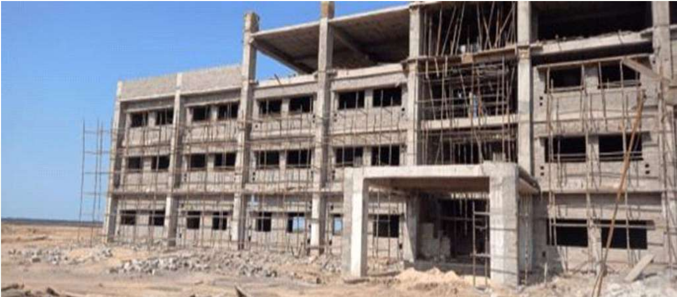
NACP construction activity
