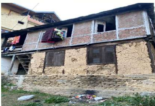
Vertical stiffness irregularities-Kullu, Himachal Pradesh
