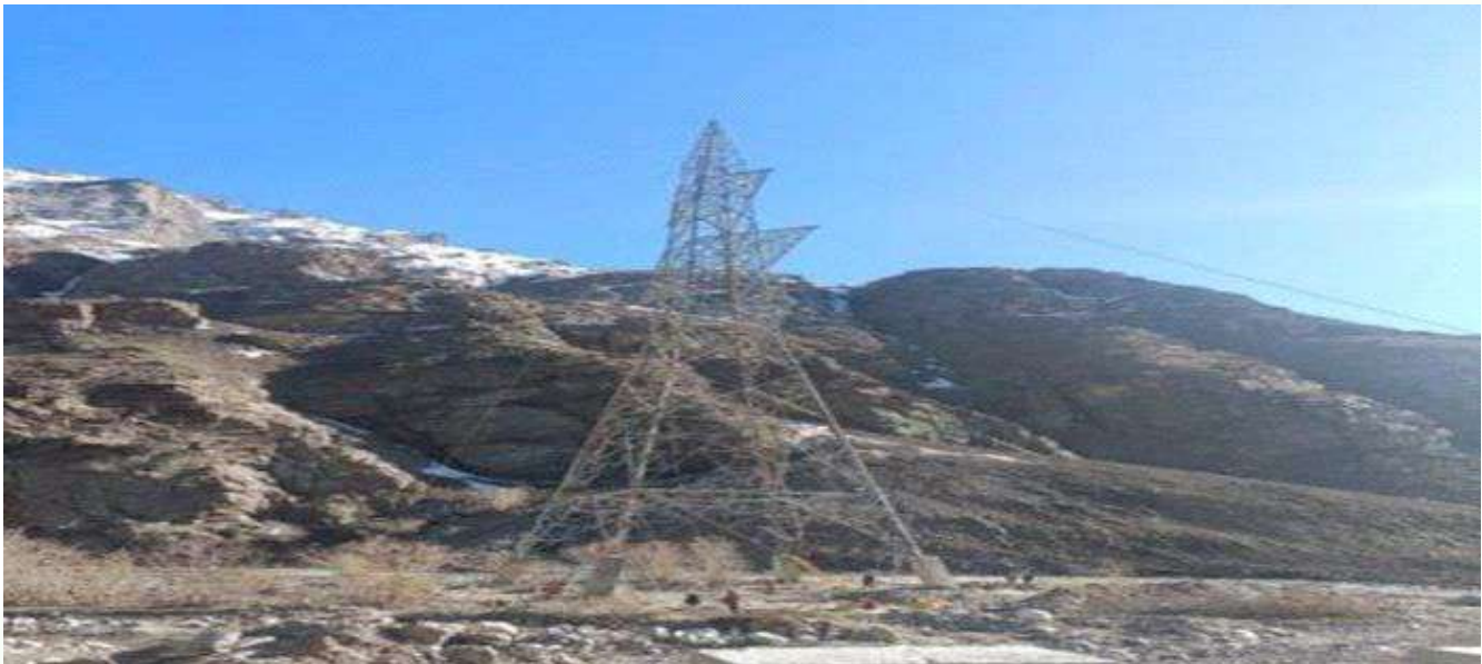
(Power Transmission line to Nubra and Zaskar)
