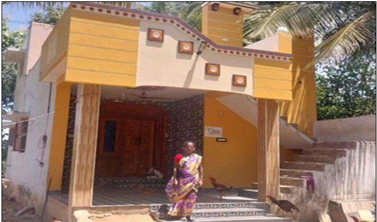
Construction of houses under PMAY (Urban)
