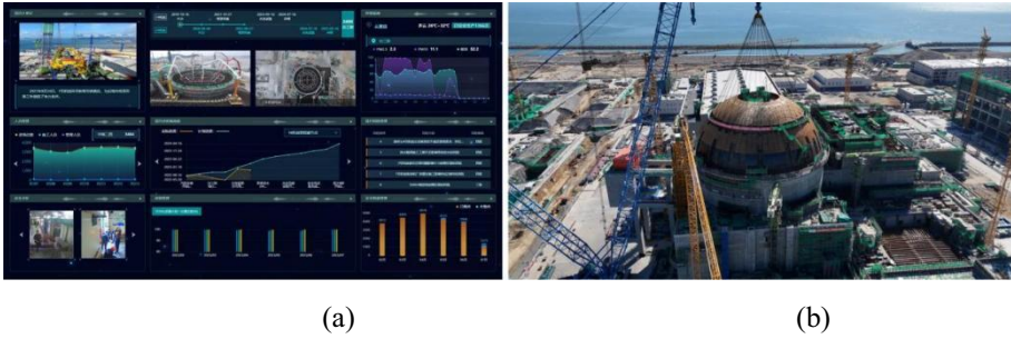
Fig. 3. Application of AI-Based Intelligent Analysis Technology in Nuclear Power Construction at the Xudapu Nuclear Power Project(a. Smart Construction Management Platform of the Xudapu Nuclear Power Project;b.Construction Site of the Reactor Building for Unit 3)
