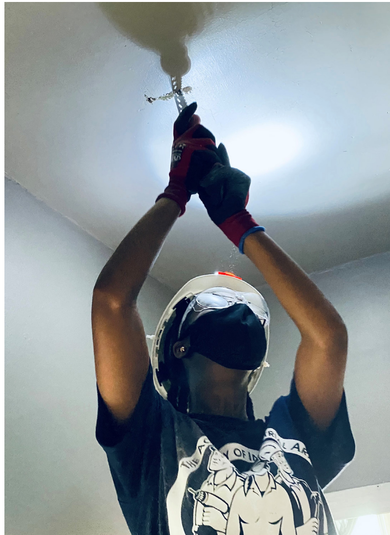
A female student at The Academy of Industrial Arts works on an electrical job.
